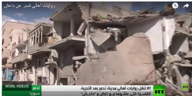
Figure 143 Civilian infrastructure destroyed by IS
