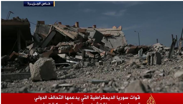
Figure 23 Material damage in Al Shaddadi after the withdrawal of IS members
