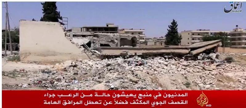
Figure 38 Material destruction caused by US-led coalition air strikes in Manbij
