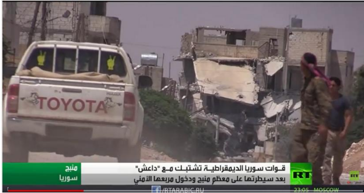
Figure 112 Material damage as result of the US-led war against IS
